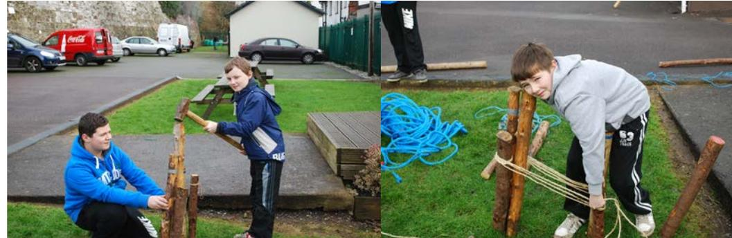
As a rule of thumb: Pickets should be positioned in the ground approx. 3 times the height from which the main rope leaves the structure. i.e. if the main rope passes over the legs at 2m above the ground then the pickets should be 6m from the base of the legs.
